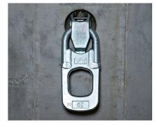
The HALFEN Recovery anchor system is a cast-in DEHA KKT Stainless steel spherical head lifting anchor, load class 20,0 on which a freely pivoting standard lifting link is attached. The lifting link is similar to the type used for moving precast concrete elements. A securing bolt is provided to prevent unintentional removal of the lifting link.
