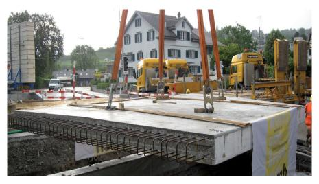
It is inevitable that elements sometimes need to be manoeuvred over critical areas and facilities. The failure of an anchor here can have devastating consequences. Even with correct calculation, deviant material quality can still constitute the critical weak spot. Anchors are subject to further stress especially from dynamic loads (shock factors). Impact strength and elongation at failure are both critical here. Selecting high quality raw material is therefore of the uppermost importance.
