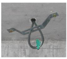
Cable loop installed in a lift shaft
